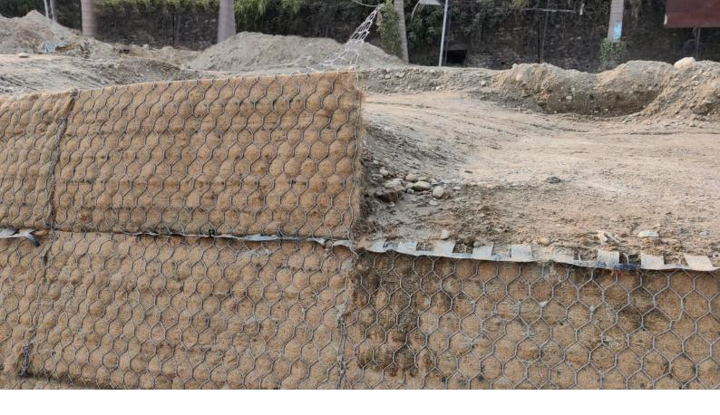
In high RSWs, a 'Green' Tailmesh sloped wall is used on top of a vertical Gabion Fascia RSW to provide a stable structure. Below is an illustrative design showing typical details of a 'Green' Tailmesh Gabion Sloping Fascia RSW.
